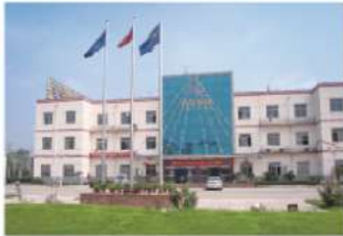
● 光事业部 Building of Optical Division
